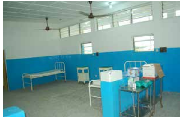
The renovated female surgical ward of Minna General Hospital by Minna Branch of Fidelity Bank
